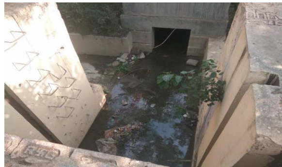
Figure 5: Khyber Pass Drain
